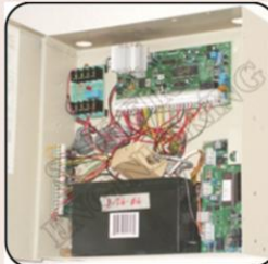
Fire Alarm System Battery
